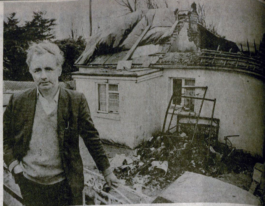
A weary looking Mr. O'Riordan at his gutted home in Carrigparson.
